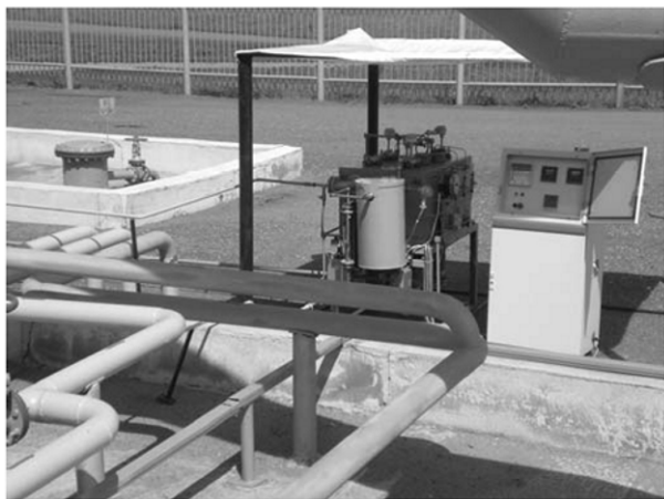
Fig. 2. Pilot unit for APG desulfurization on flare line.
